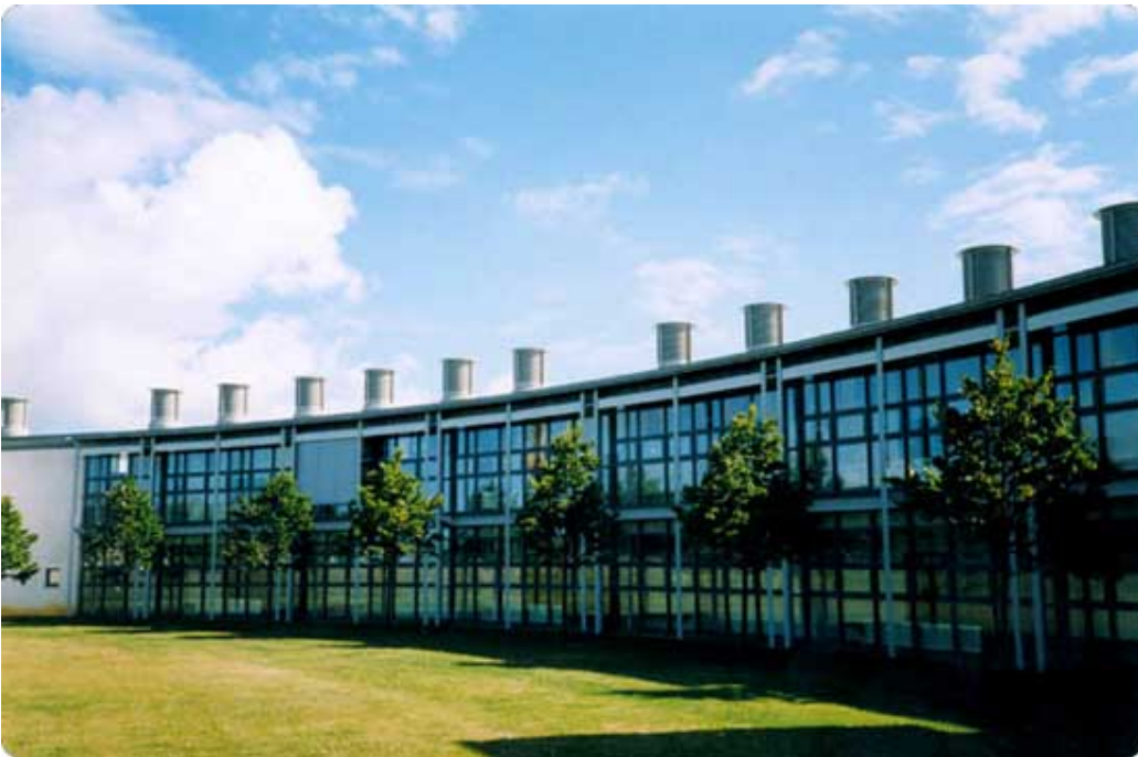
Figure 3. Examples of installed Monodraught windcatchers in the UK: 1000 mm square system at Imperial College (above) and 1000 mm circular-cylindrical windcatchers at St Annes School, Jersey (below)
