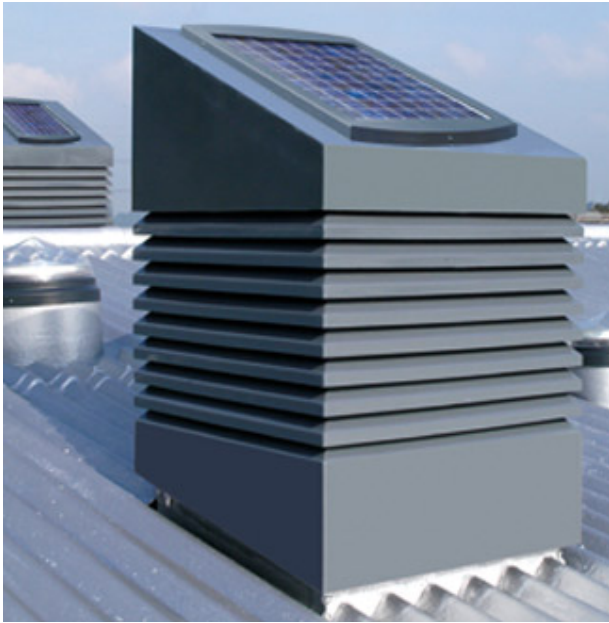
Figure 4. An installed system of solar-boosted windcatchers from Monodraught.
